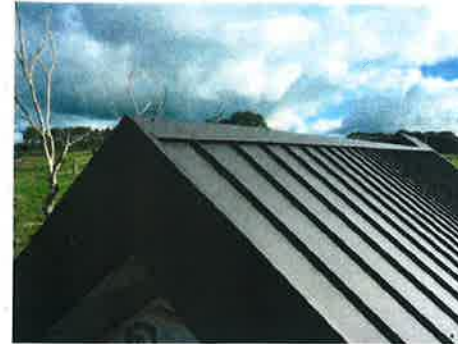
1. MONUMENT COLORBOND KLIP LOK ROOF SHEETING
